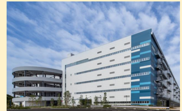
【Low temperature transportation and delivery center (South Tokyo area)】
